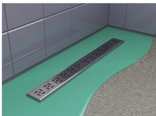
4. Cover the flange and the surrounding area with an insulating foil in a liquid form.
