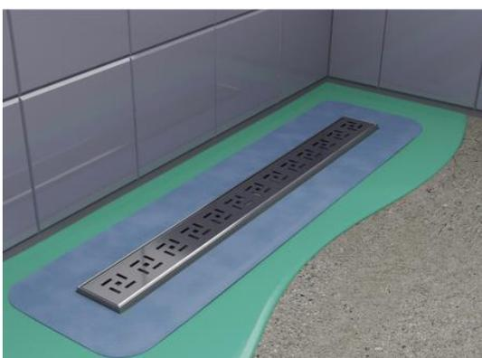
5. Apply the sealing membrane in position on the freshly applied liquid foil.
