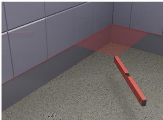
1. Set the level of the finished shower floor surface and mark it on the wall in the area where the channel will be fitted (allow for the slope of the shower surface)
