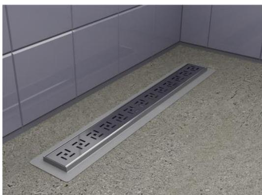
3. Fill the space under and around the channel with screed or a similar product to the level of the flange.
